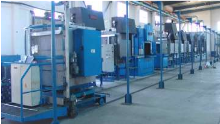
Aichelin furnaces for bainite treatment in RKB T3 Plant
